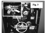
Water heater drain plug location
